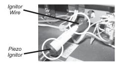
**17)** Disconnect the ignitor wire from the Piezo Ignitor and connect it to the DC Sparker.
